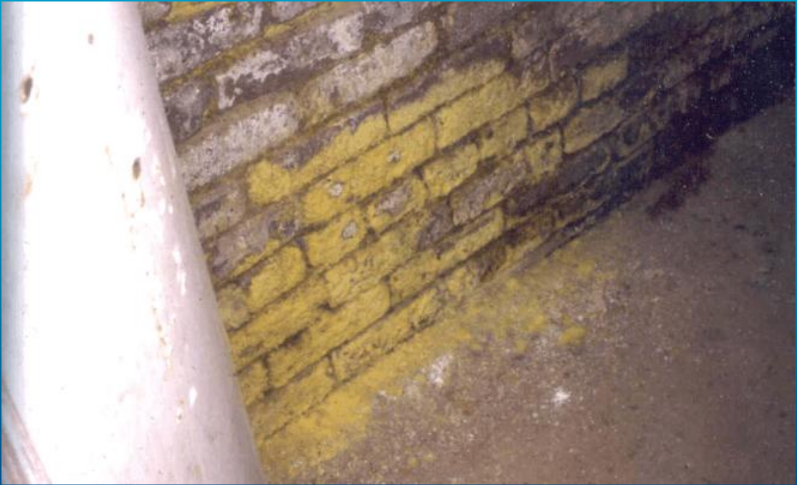
Yellow chromate crystals on inside of basement wall in 1990s prior to cleanup
